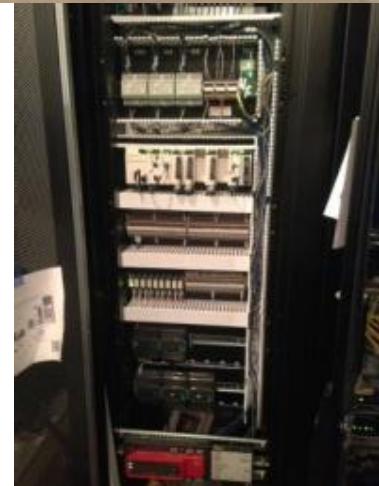
Site microgrid controller + DSO hardware
