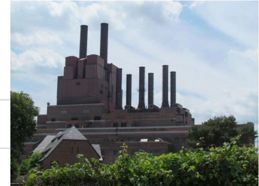
Marysville Power Plant, Commissioned 1922, Decommissioned 2001, Imploded Nov. 2015 https://www.wikiwand.com/en/Marysville_Power_Plant
