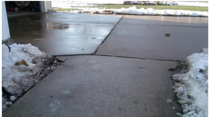
HDF-2019-9944-NEP 670 Starfield Cement Repairs AFTER
