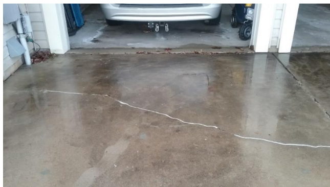
HDF-2019-9944-NEP 670 Starfield Cement Repairs AFTER
