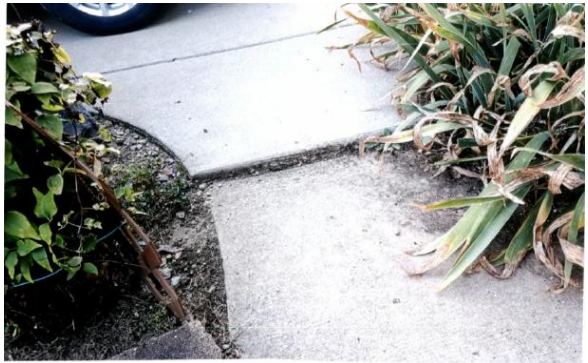
HDF-2019-9944-NEP 699 Vincent Step and Cement Repairs BEFORE
