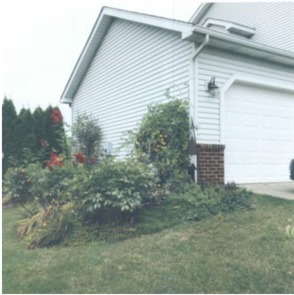
HDF-2019-9944-NEP 10168 Honeycomb Ct Door BEFORE
