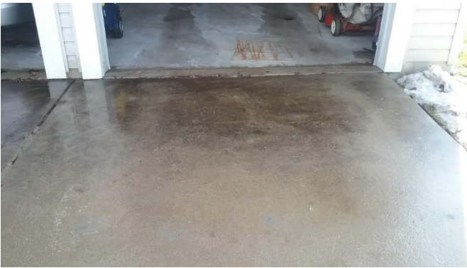
HDF-2019-9944-NEP 670 Starfield Cement Repairs AFTER
