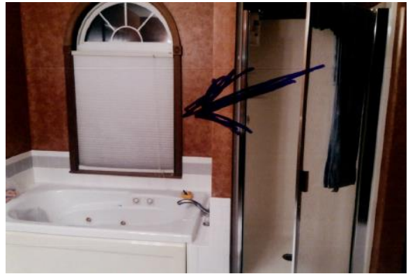
HDF-2019-9944-NEP 670 Starfield Window Repairs BEFORE
