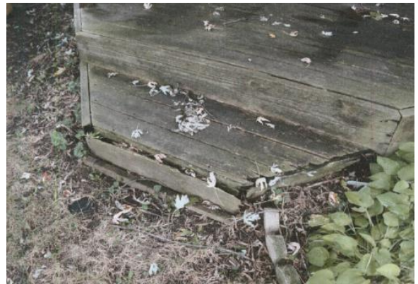
HDF-2019-9944-NEP 10369 Barbara Deck Repairs BEFORE
