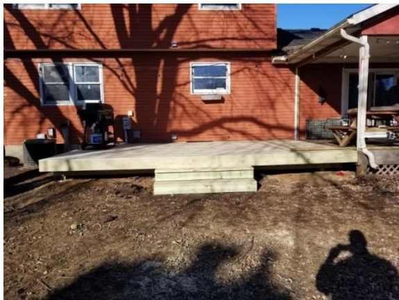
HDF-2019-9944-NEP 10369 Barbara Deck Repairs AFTER
