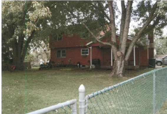
HDF-2019-9944-NEP 10369 Barbara Deck Repairs BEFORE
