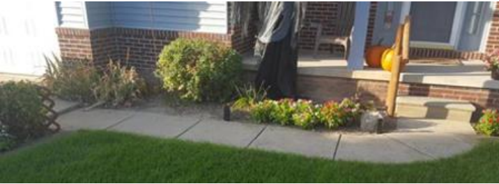
HDF-2019-9944-NEP 699 Vincent Step and Cement Repairs BEFORE
