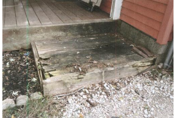
HDF-2019-9944-NEP 10369 Barbara Deck Repairs BEFORE
