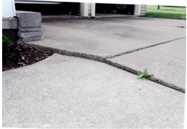
HDF-2019-9944-NEP 670 Starfield Cement Repairs BEFORE
