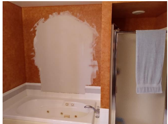
HDF-2019-9944-NEP 670 Starfield Window Repairs AFTER
