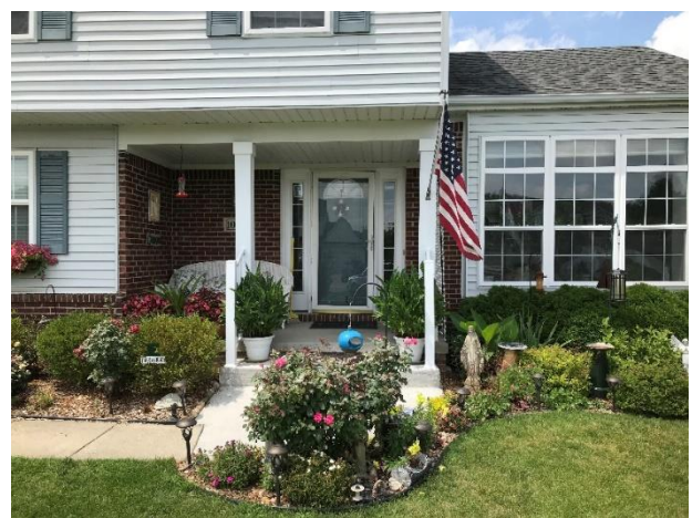
HDF-2019-9944-NEP 10168 Honeycomb Ct Cement/Handrail Repairs AFTER
