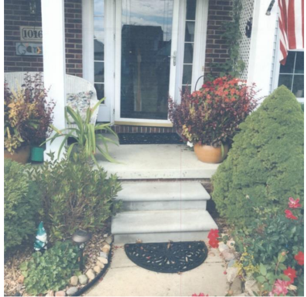
HDF-2019-9944-NEP 10168 Honeycomb Ct Cement/Handrail Repairs BEFORE
