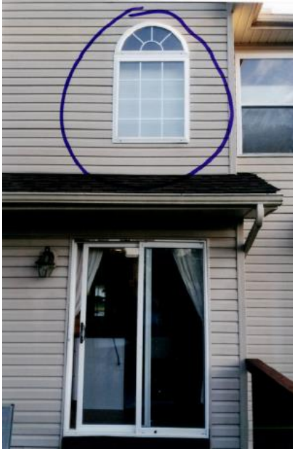
HDF-2019-9944-NEP 670 Starfield Window Repairs BEFORE
