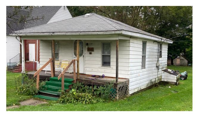
Before: This home had very old aluminum siding. It did not have any insulation underneath, making the home very cold in the winter. Most of the wood trim around the windows had rotted away and left large gaps, leaving the home vulnerable to further damage and deterioration.
