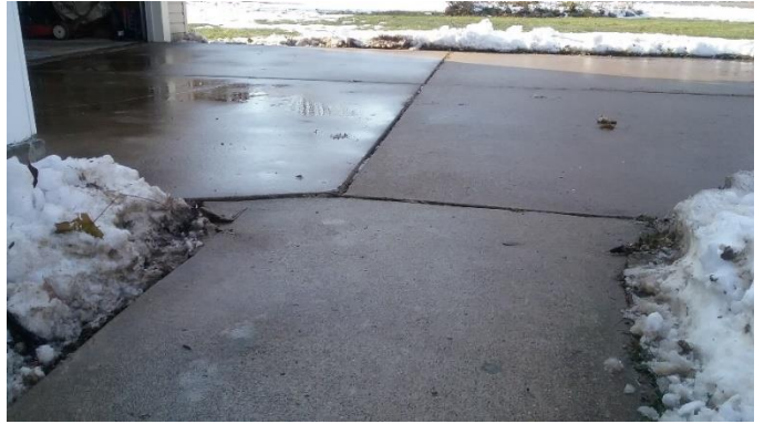
HDF-2019-9944-NEP 670 Starfield Cement Repairs AFTER
