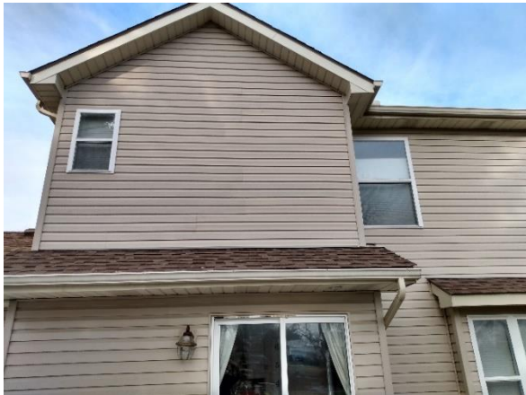
HDF-2019-9944-NEP 670 Starfield Window Repairs AFTER
