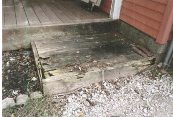
HDF-2019-9944-NEP 10369 Barbara Deck Repairs BEFORE
