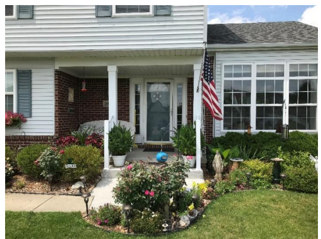
HDF-2019-9944-NEP 10168 Honeycomb Ct Cement/Handrail Repairs AFTER
