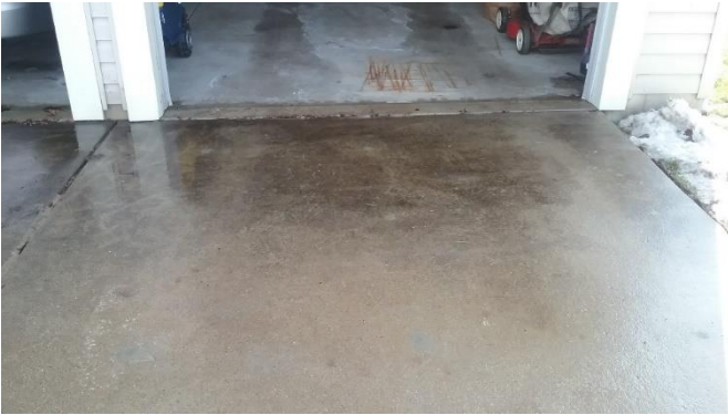
HDF-2019-9944-NEP 670 Starfield Cement Repairs AFTER
