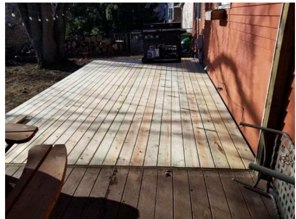
HDF-2019-9944-NEP 10369 Barbara Deck Repairs AFTER
