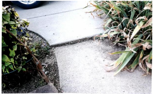
HDF-2019-9944-NEP 699 Vincent Step and Cement Repairs BEFORE
