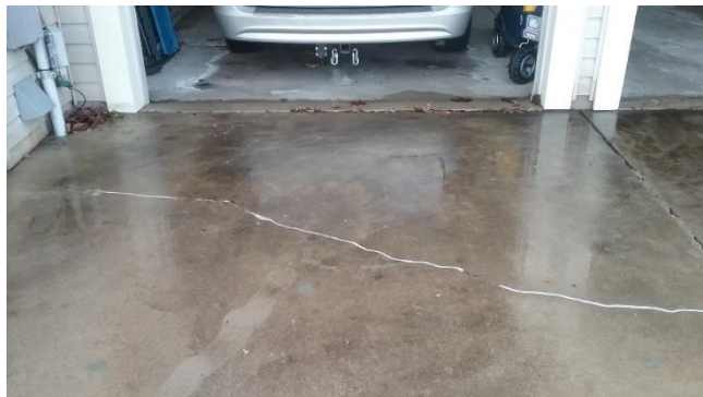
HDF-2019-9944-NEP 670 Starfield Cement Repairs AFTER
