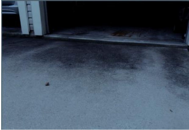
HDF-2019-9944-NEP 670 Starfield Cement Repairs BEFORE
