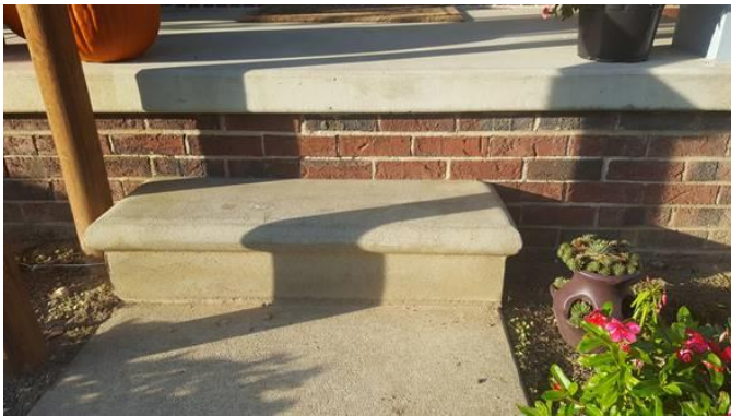
HDF-2019-9944-NEP 699 Vincent Step and Cement Repairs BEFORE
