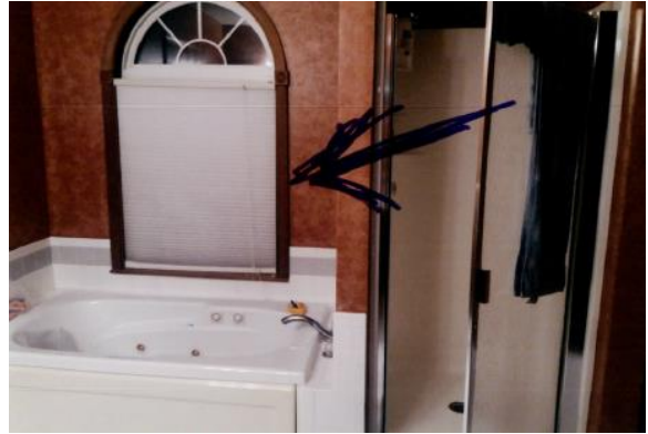
HDF-2019-9944-NEP 670 Starfield Window Repairs BEFORE
