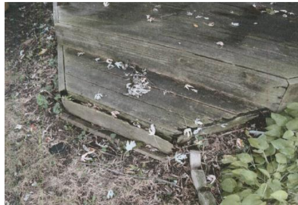
HDF-2019-9944-NEP 10369 Barbara Deck Repairs BEFORE
