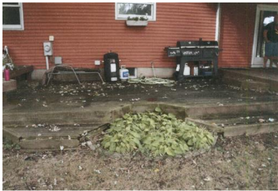
HDF-2019-9944-NEP 10369 Barbara Deck Repairs BEFORE
