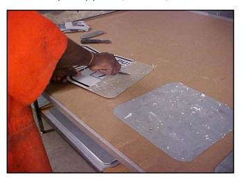
By utilizing skilled labor, MSI's "GREEN" Sign Restoration process applies heat that removes worn out reflective sheeting material from old signs without damaging the corrosion-resistant coatings on the metal. The signs are manually peeled and scraped, cleaned, and a chemical process is used to clean the blank. New reflective sheeting materials are applied, providing motorist more notice and increased safety.
