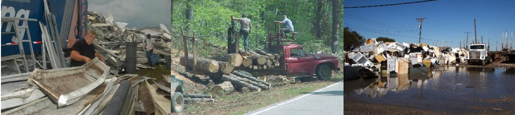
L-R: metal debris being separated for recycling; log salvagers reducing the volume of vegetative debris that must be ultimately disposed of; metal appliances being recycled.
