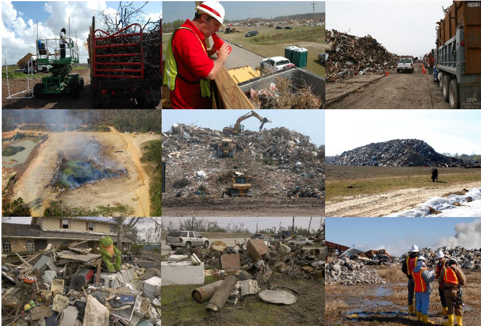
L-R, Top Row: TDSR Site inspection station temporary viewing platforms (mechanical and constructed); inspection station without viewing platform (using pickup truck as a base); Middle Row: aerial view of TDSR Site for burning operations with adequate buffer zones around the perimeter; piles of C&D debris waiting to be processed and then disposed of; Bottom Row: unsorted debris piles along roadways make recycling efforts more difficult – but not impossible; fires are always a threat at TDSR Sites, making adequate ingress / egress and roadways critically important for fire suppression purposes.
