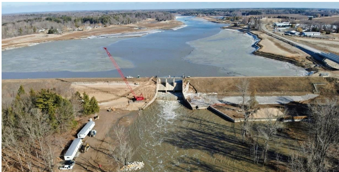
Tobacco River flow being restored to its normal course as repair progressed at the Edenville Dam, 2021
