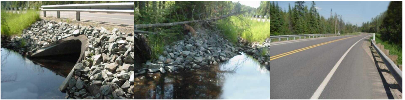
Photos L-R show completed culvert replacement, bank stabilization and road resurfacing.
