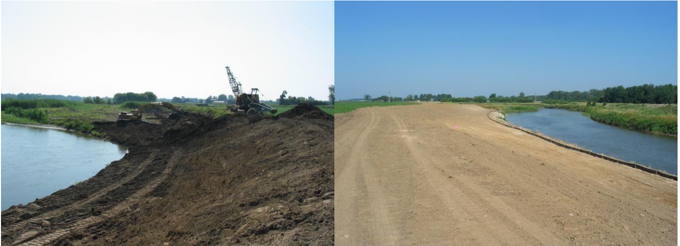
Photos L-R: A section of the dike under construction in Saginaw County; a reconstructed section of the dike, before final grading and reseeding. The new dike is constructed to modern standards with a wider course, 1:4 slope setbacks, and a series of detention areas and flood spillways to accommodate excessive flow.
