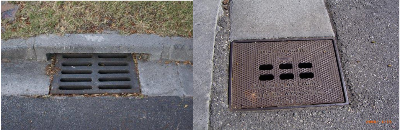
Photos L-R: Pre-construction – non-restricted catch basin cover. Post Construction – example of one of the 2,300 restricted catch basin covers installed throughout the City of Wyandotte.
