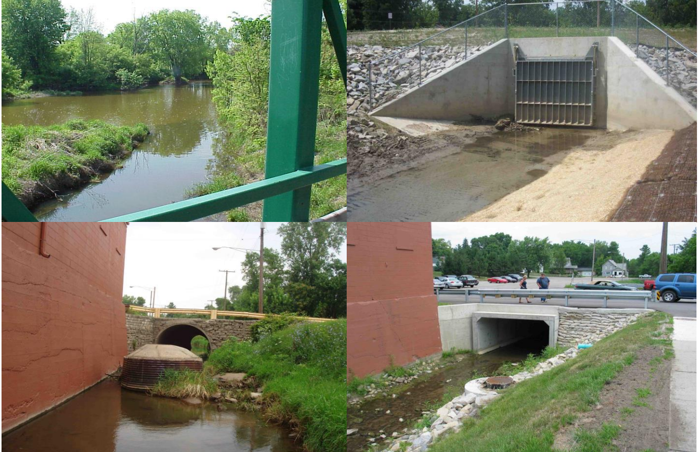
Top Row L-R: Pre-construction – Moore Drain outlet to Cass River with no outlet structure; Post-construction – Moore Drain outlet to Cass River (new) with backflow flap gate; Bottom Row L-R: Pre-construction – Moore Drain downtown parking lot culvert (inadequate); Post-construction – Moore Drain downtown parking lot culvert (improved).
