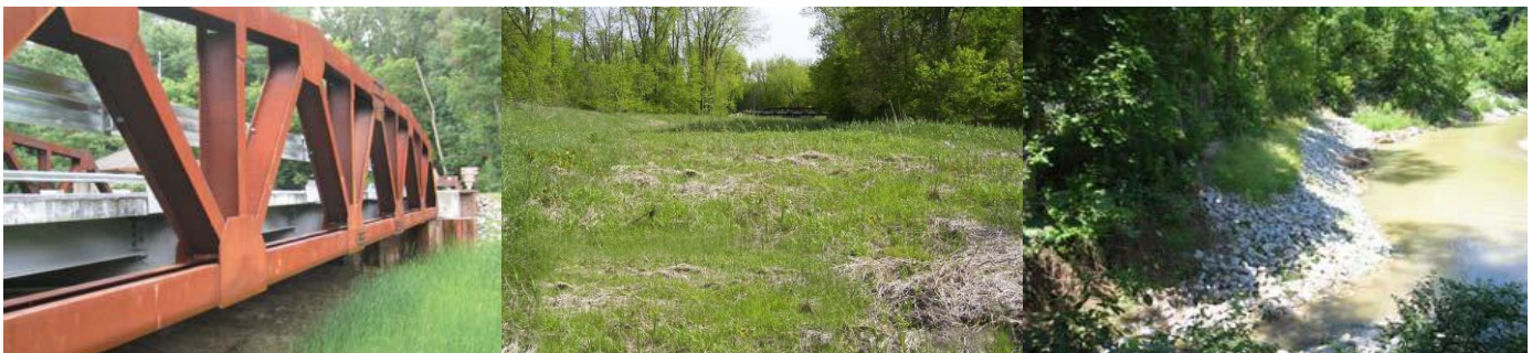
Photos L-R: The New Union Street Bridge replaced an undersized culvert to improve water flow; the emergency floodway with the Union Street Bridge in the background; rip-rap slope protection in the Intercounty Drain.
