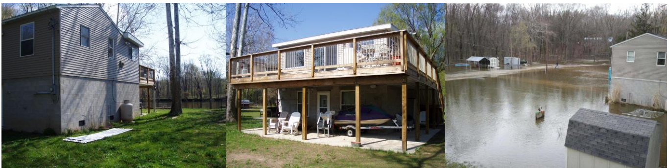
Photos L-R: The west and south sides of the elevated home; note the proximity of the Muskegon River. The elevated home during the late April-early May 2011 flooding of the Muskegon River. The home was surrounded by floodwater but suffered minimal damage.
