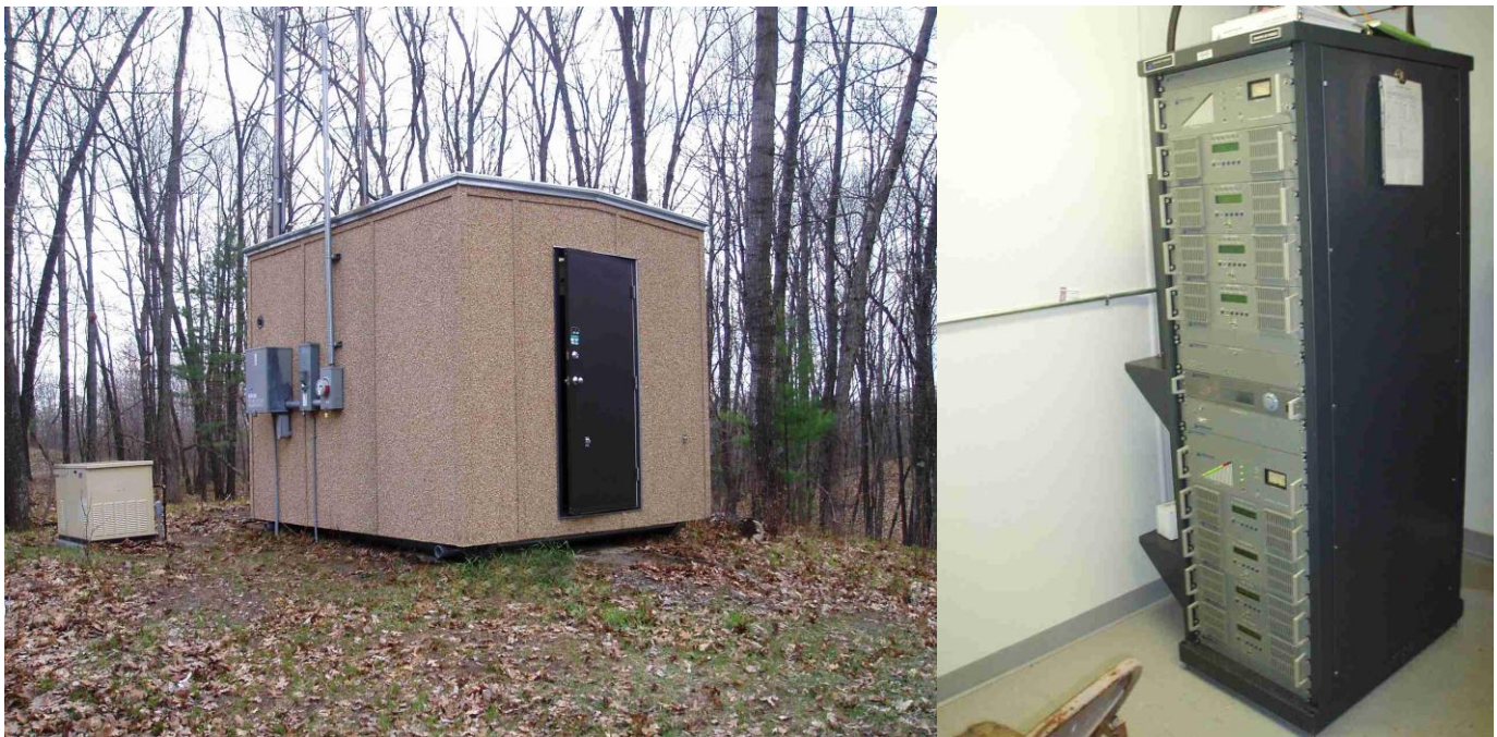
Photos L-R: Transmitter equipment building with back-up generator; transmission equipment inside transmitter equipment building.
