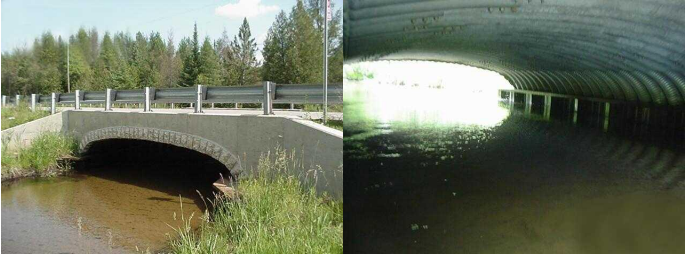
Photos L-R show the new 22-foot box culvert which replaced an inadequate twin culvert system. Concrete headwalls were also installed and stream bank stabilization measures, such as rip-rap, were taken.
