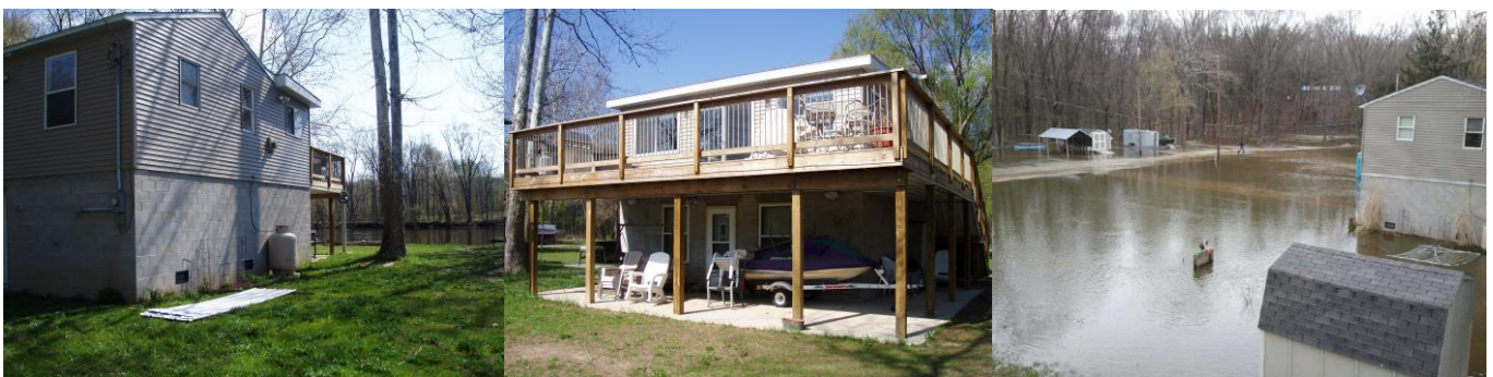
Photos L-R: The west and south sides of the elevated home; note the proximity of the Muskegon River. The elevated home during the late April-early May 2011 flooding of the Muskegon River. The home was surrounded by floodwater but suffered minimal damage.
