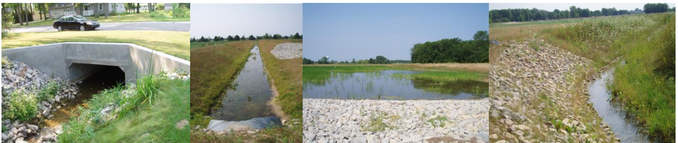
Photos L-R: View of new culvert with wing walls; improved drain channel with rip-rap overflow; view of detention pond; inlet channel with erosion control.
