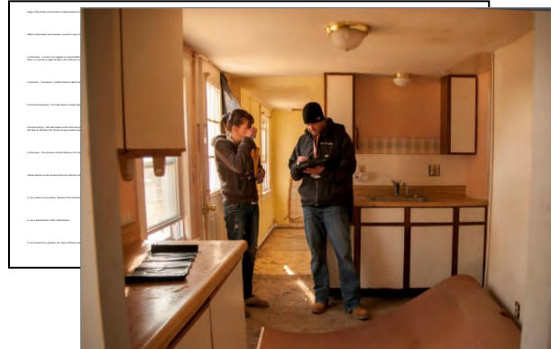
A FEMA inspector speaks with resident of a home damaged by Hurricane Sandy during an on-site inspection in New Jersey.
