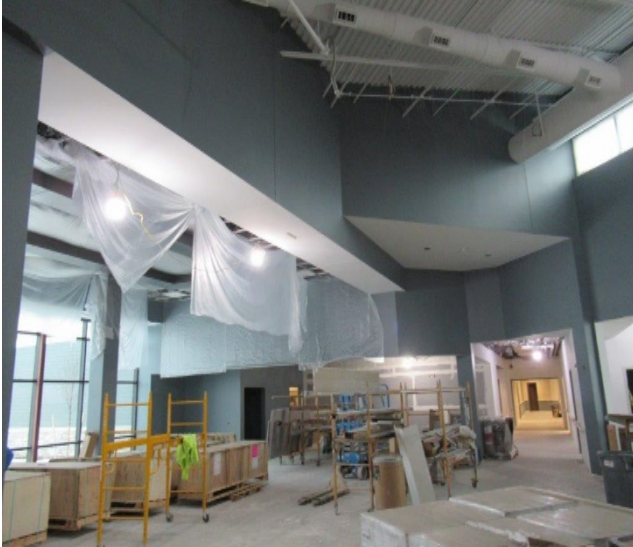
CC Main Lobby - 1/7/21
