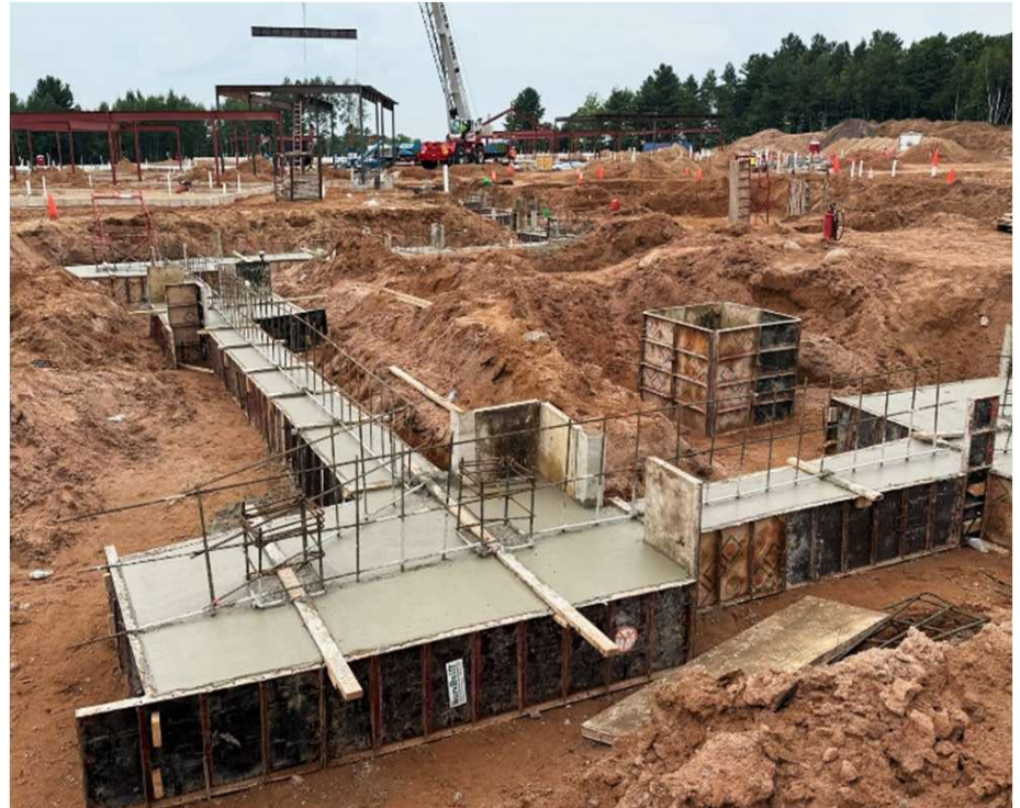
Footing/Foundation Wall C1 8/3/2026
