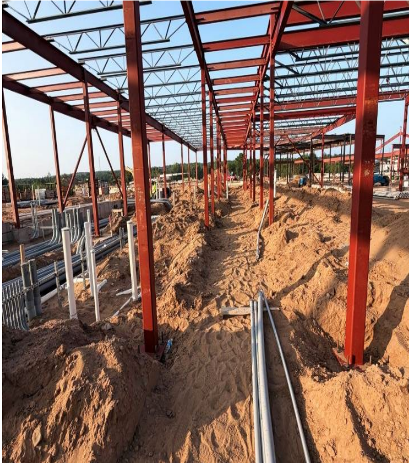
Steel Erection C2 8/3/2026
