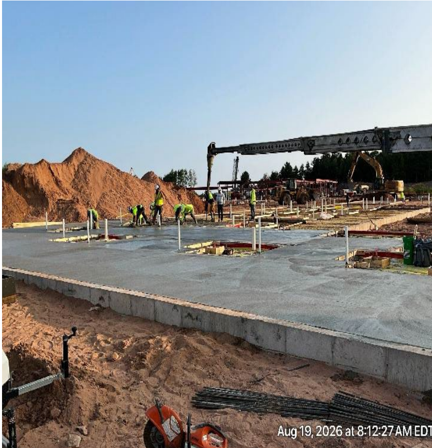
Slab on grade – N3 8/19/2026
