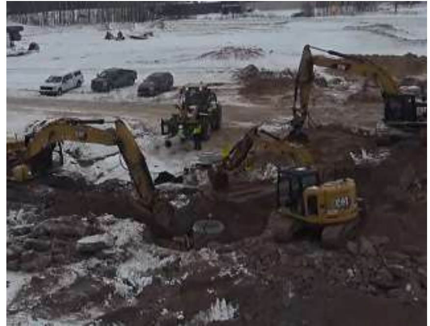
Installing Storm Pipe/Structure along Perimeter Road
