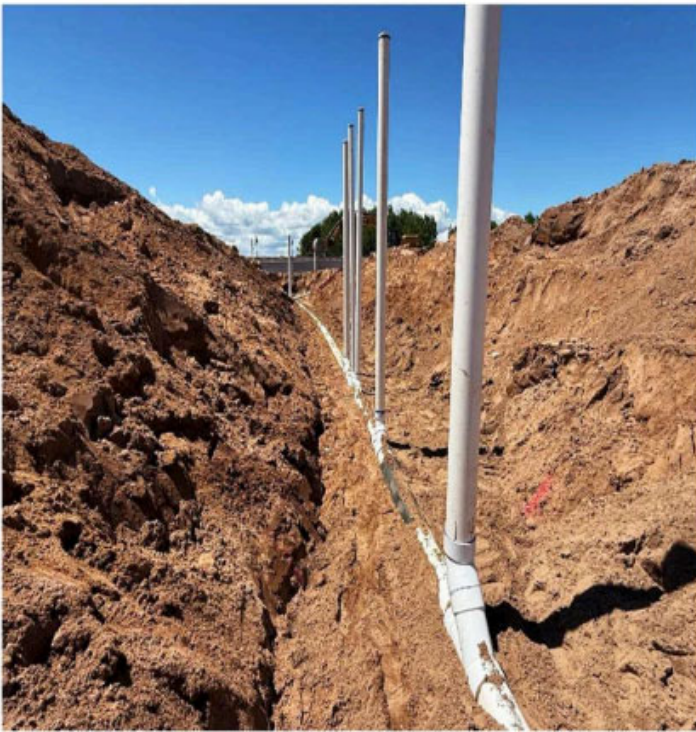
Installing Sanitary Connection at Community Center 7/2/2026
