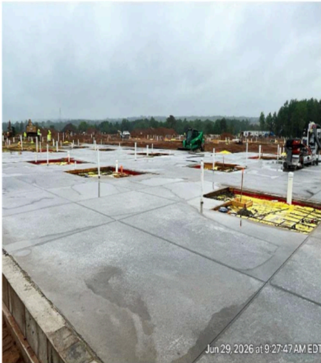
Slab on Grade N1 6/29/2026
