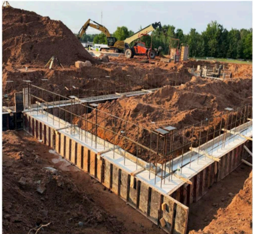
Footing/Foundation Wall N3 6/29/2026
