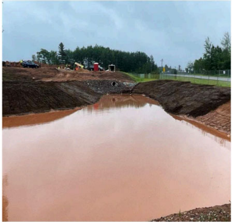
Retention Pond Shaping 6/26/2026
