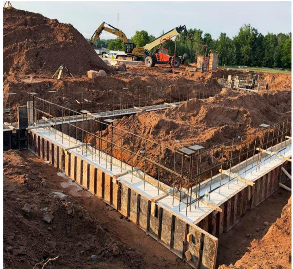
Footing/Foundation Wall N3 6/29/2026
