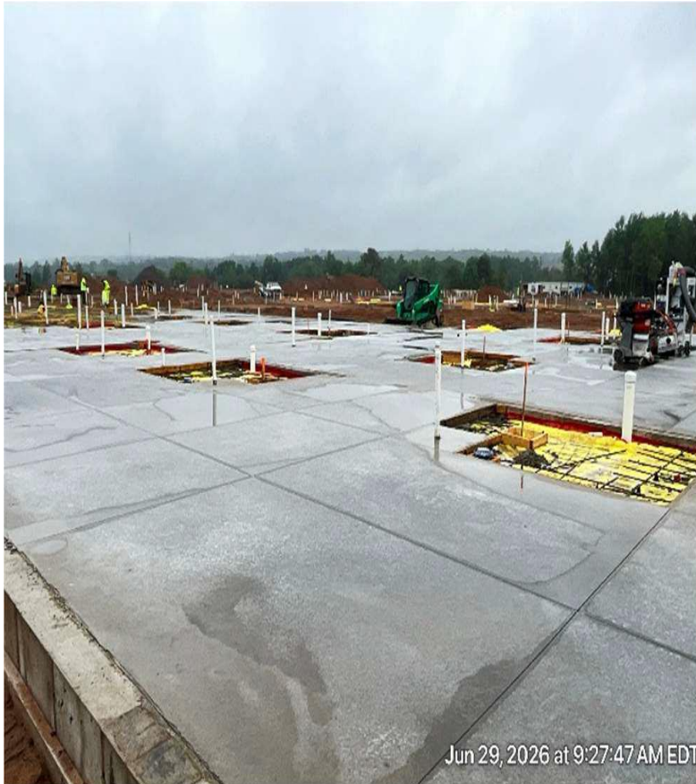
Slab on Grade N1 6/29/2026
