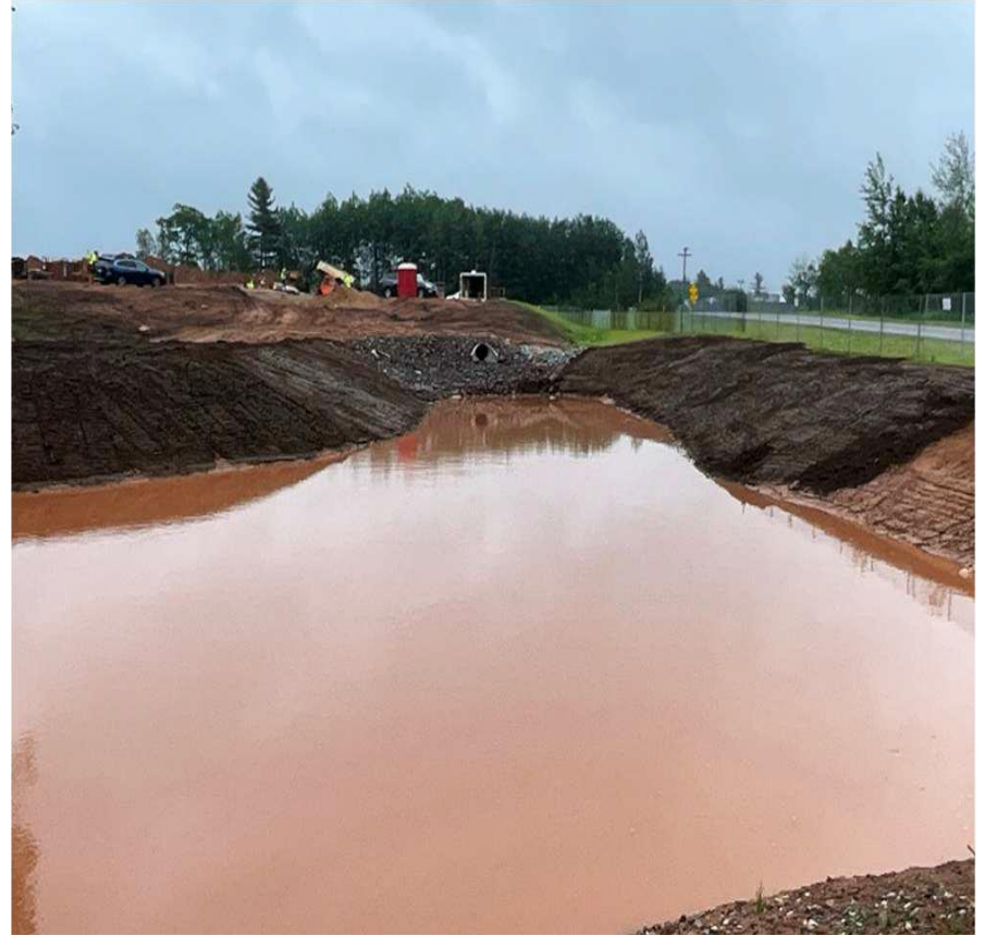
Retention Pond Shaping 6/26/2026
