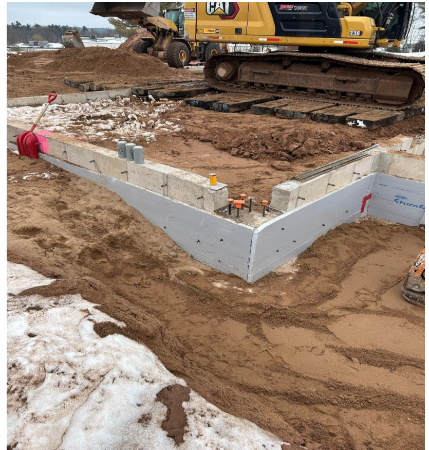
Foundation Insulation
