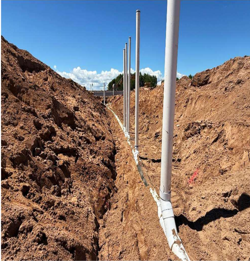
Installing Sanitary Connection at Community Center 7/2/2026
