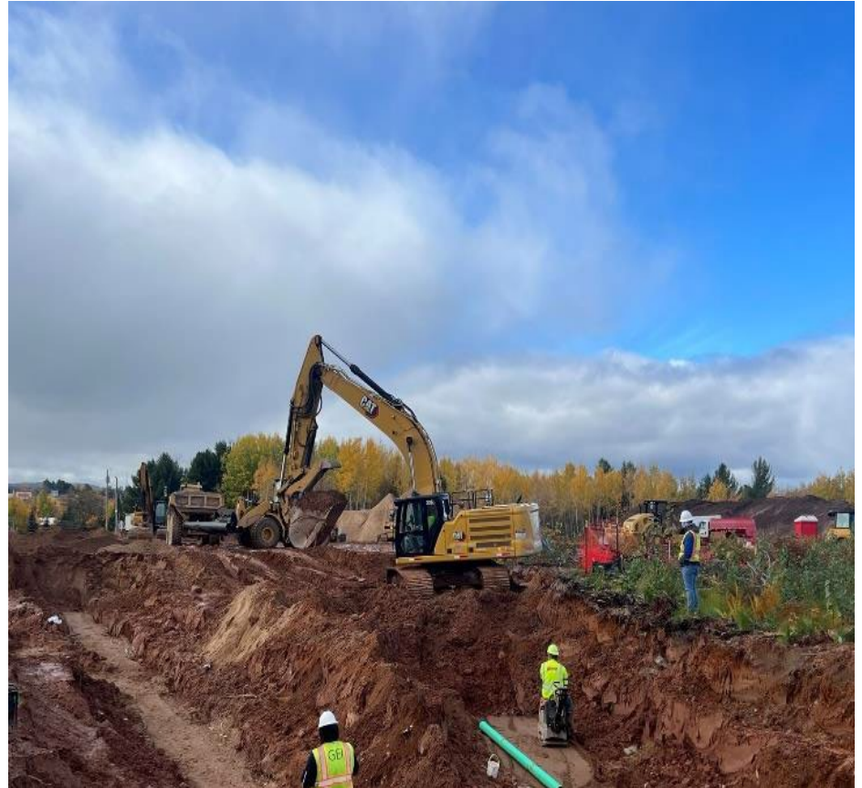
Water Main Pipe installation 10/24/2025
