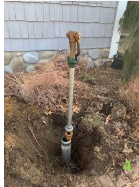
Exposing the drop pipe and interior portion of the pitless adapter.
