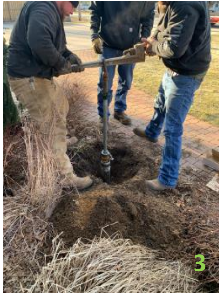
Pulling the drop pipe by hand.
