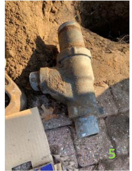
Well head and pitless adapter casing removed; well filled with Bentonite.
