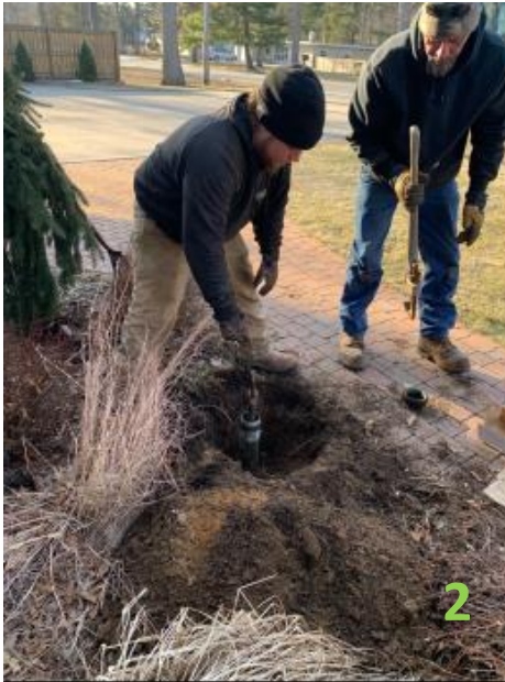
Pulling bail attached to well drop pipe.
