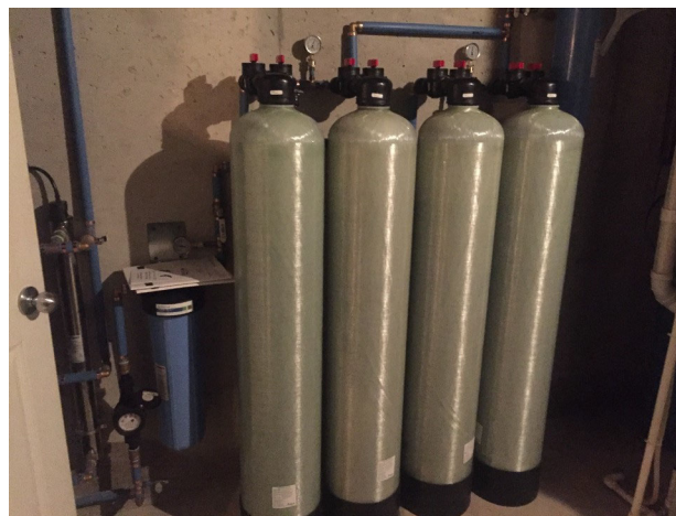
Whole-house filters like the one above have been installed in affected homes.
