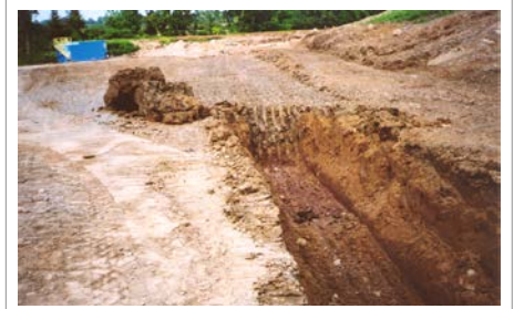
Perimeter Clay Cutoff Wall
