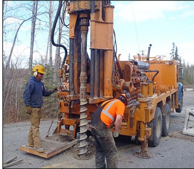
Install New Monitoring Wells
