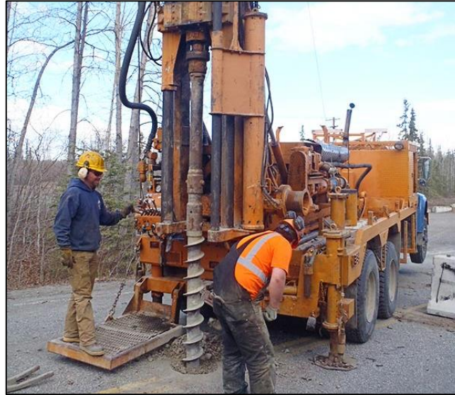
Install New Monitoring Wells
