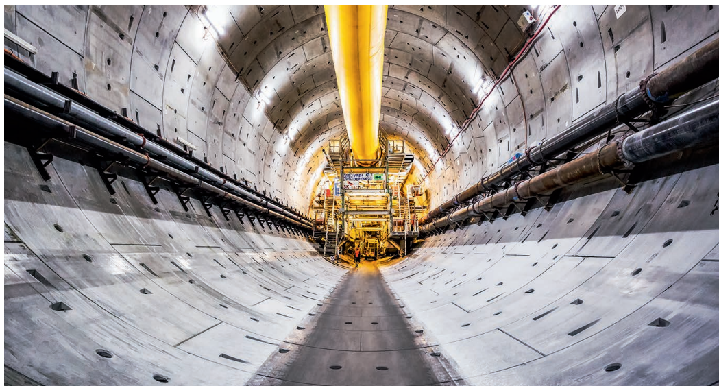
Figure 5: Precast concrete lining in the completed Eurasia Tunnel project in Istanbul. (Source: Herrenknecht)
