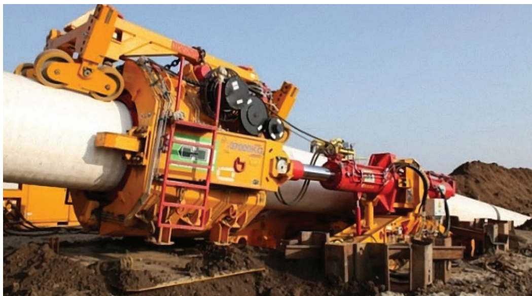
Figure 6: A pipe thruster pushing pipe.
