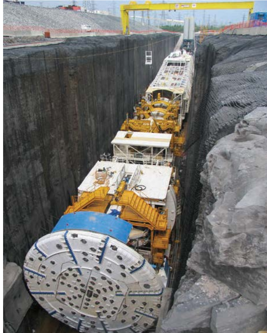
Niagara tunnel portal (45 ft diam. TBM)
