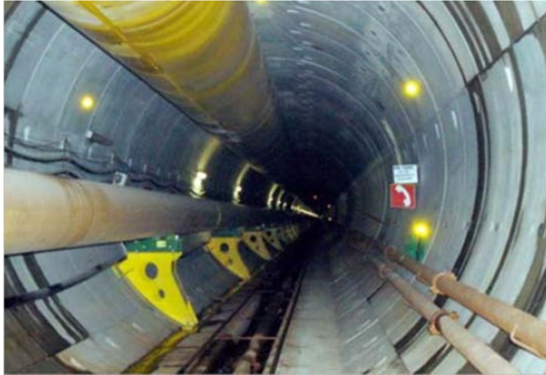
Gastau tunnel (17.5 ft internal diameter)
