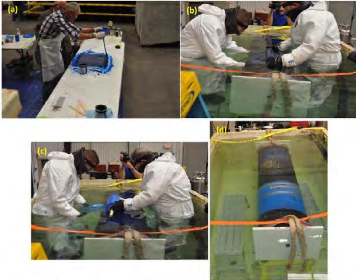
Figure 12: Application of patch repair at Area "A." Photographs show (a) impregnation of 12" x 12" fabric with epoxy; (b) application of repair on pipe in water tank; (c) wrapping repair with stricture; and (d) completed repair.
