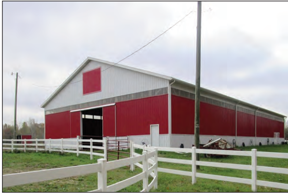
GOOD CLASS DPOLE FEEDER BARN
