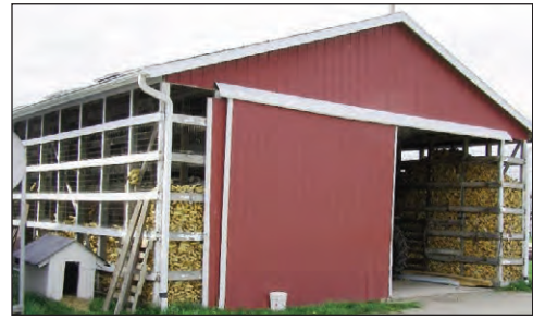
CLASS D CORN CRIB Wire-mesh-covered Exterior
