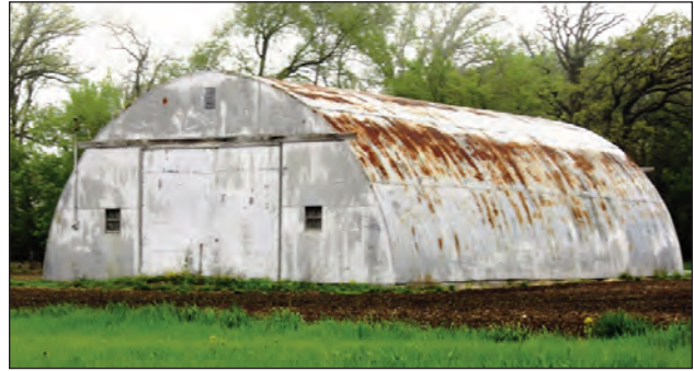
LOW CLASS S QUONSET UTILITY
