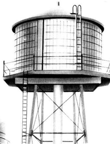
WOOD TANK ON TOWER
