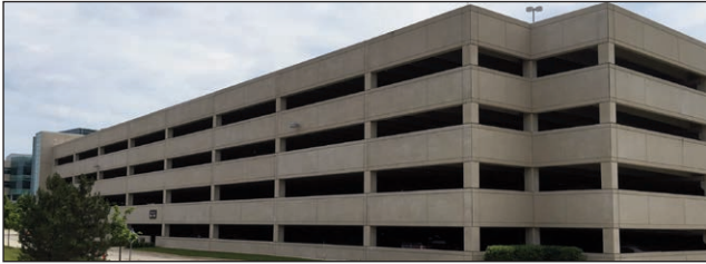
GOOD CLASS B PARKING STRUCTURE
