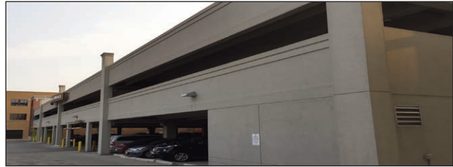
GOOD CLASS B PARKING STRUCTURE
