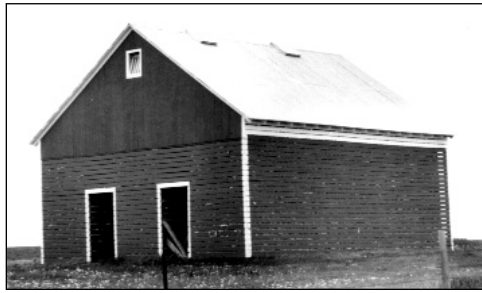
CLASS D CORN CRIB Wood-covered Exterior
